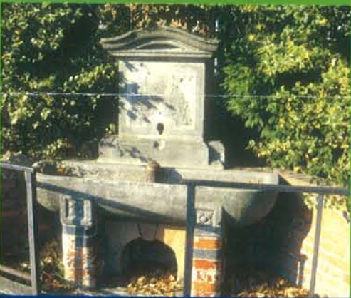
Water Trough - Fountain Lane - FP's 2 & 34
