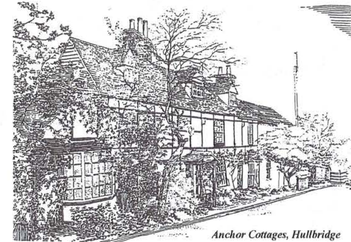
Anchor Cottages, Hullbridge
