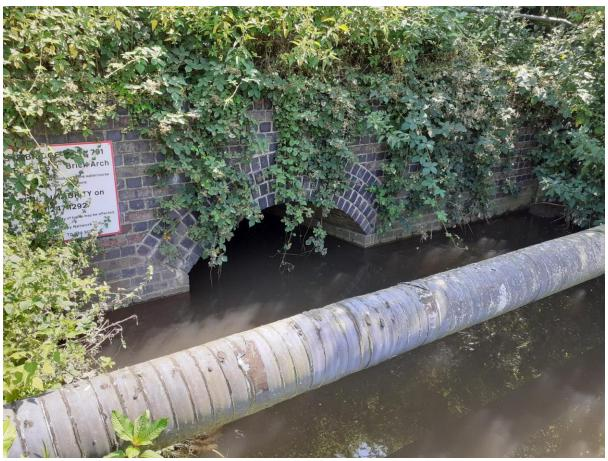
The picture above was taken in July during a dry period and shows the level of water normally present. Following rainfall it appears that culvert under the railway is not able to deal with the increase in the water flow which causes the brooks to flood the course.
