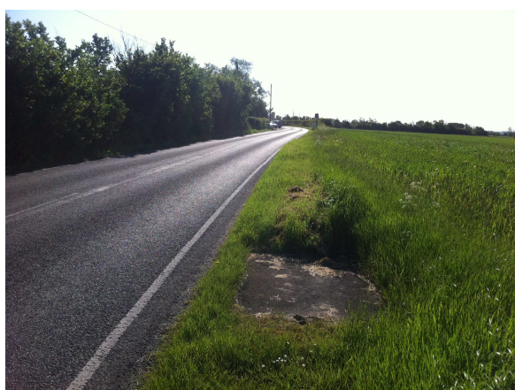
Plate 6: Westbound bus stop
