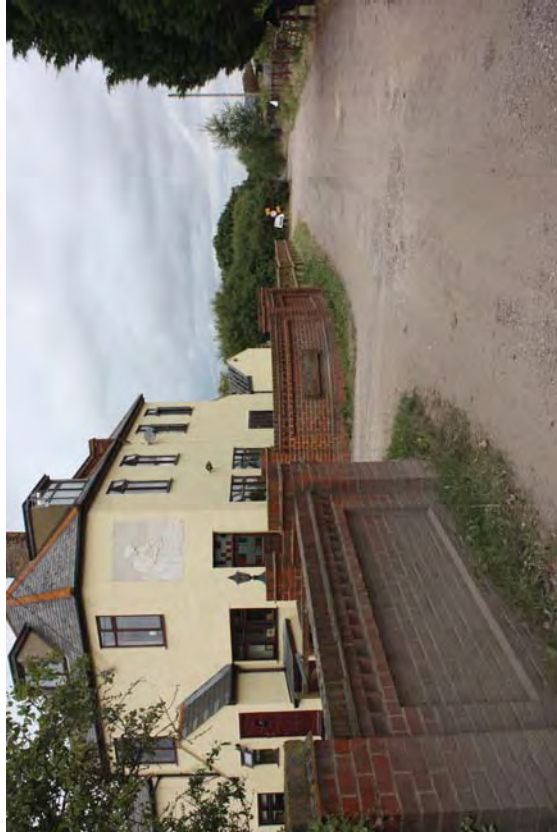
Development at Trenders Avenue Photograph 21
