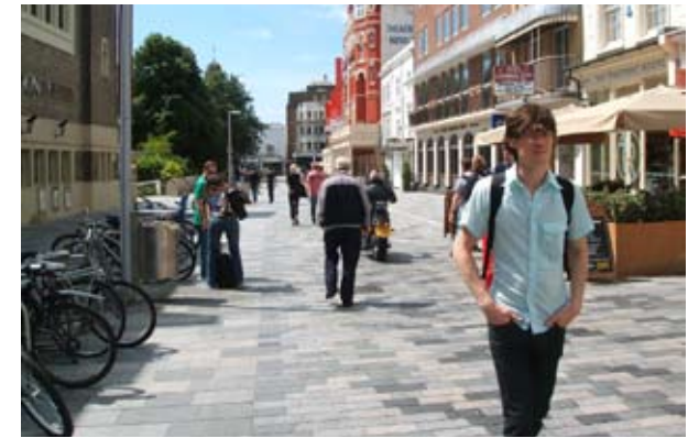
Figure 100: Shared space scheme, New Road, Brighton
