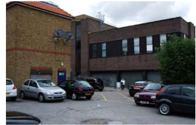
Figure 70: Rear service areas, Websters Way
