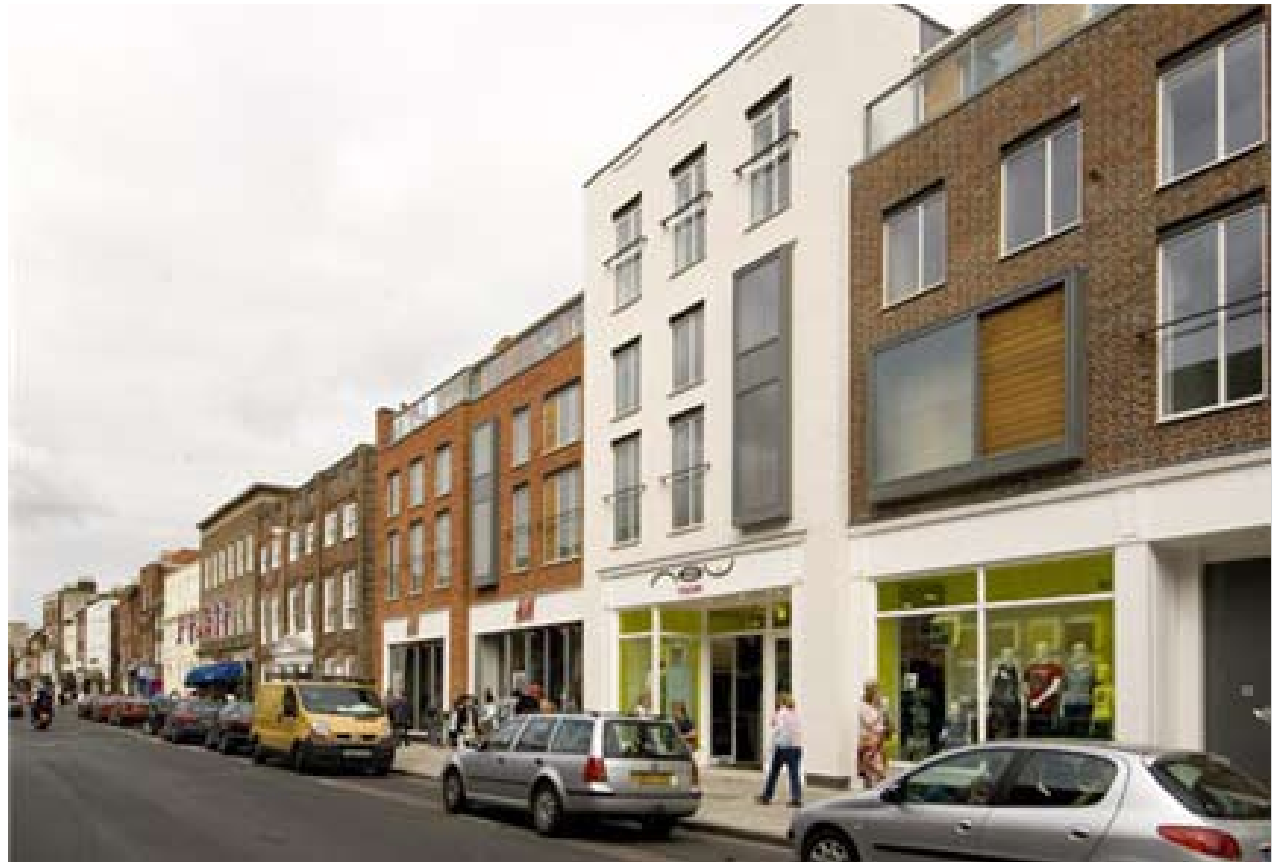
Figure 49: Potential for new retail-led mixed use development on the police station site, reflecting the grain and rhythm of the historic built form, as at Chichester
