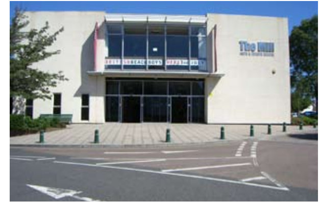
Figure 58: The Mill arts and leisure centre
