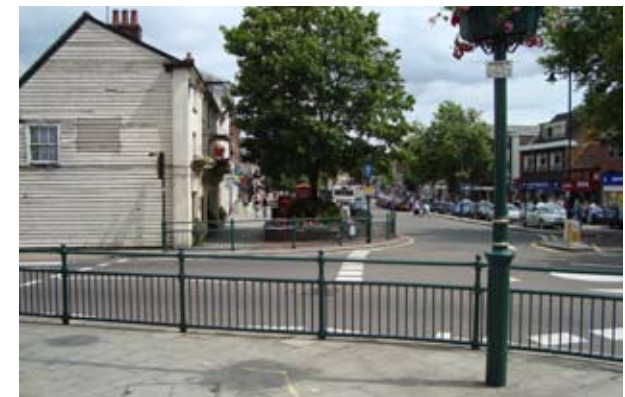
Figure 96: Guardrail at the Crown Hill / High Street junction
