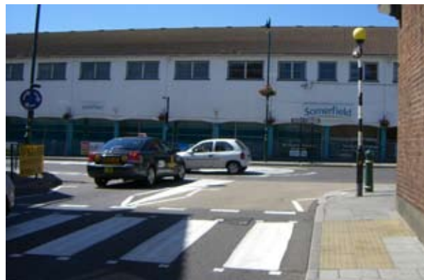
Figure 44: Somerfield store, viewed from Websters Way
