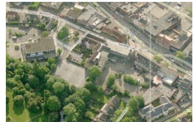
Figure 63: Area behind Bellingham Lane (source: bing.com)
