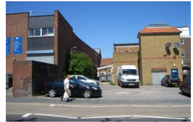
Figure 32: Exposed servicing areas on Websters Way
