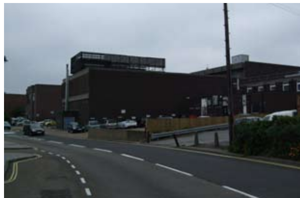
Figure 73: Rear of the former Tesco store on Websters Way
