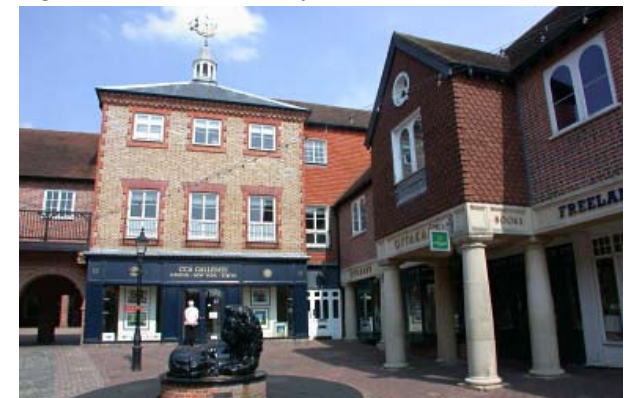
Figure 80: Mixed use retail and residential development reflecting historic character of the town, Lion & Lamb Yard, Farnham
