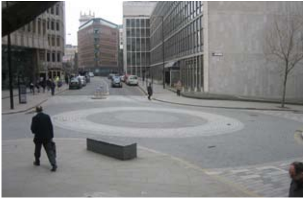
Figure 102: Junction treatments, Shoe Lane, London
