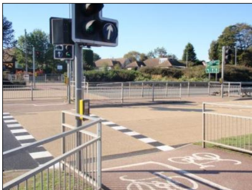
Figure 3.16 – Toucan Crossing East of Westbourne Grove
