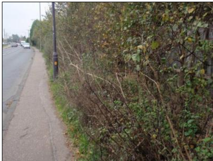
Figure 3.12 – Narrow footway on South End Road
