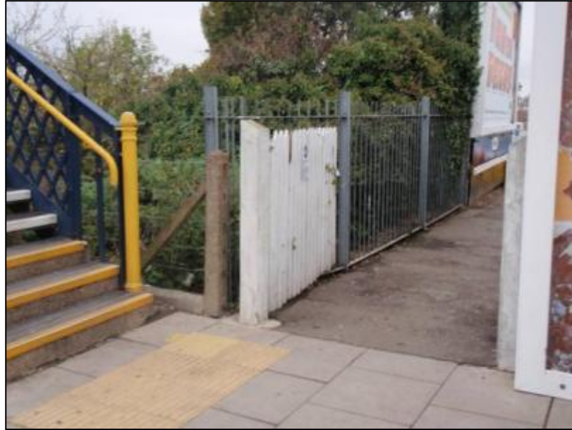
Figure 3.20 – Access to the car park on platform 1
