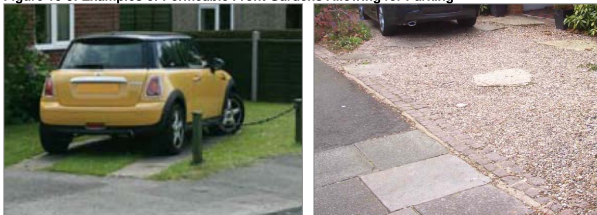
Figure 10-5: Examples of Permeable Front Gardens Allowing for Parking
