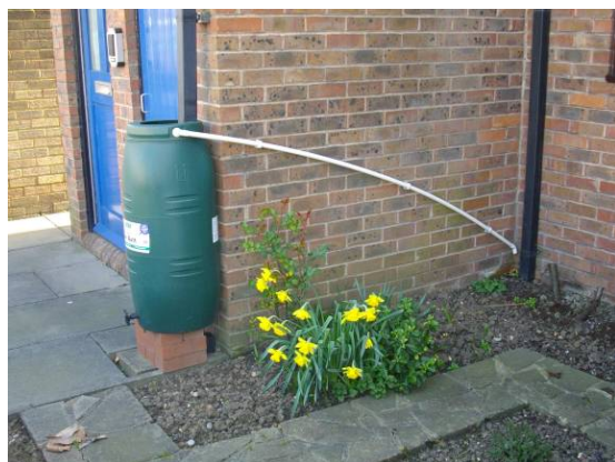
Figure 10-7: Example of a 100L Water Butt Retrofitted to Existing Development
