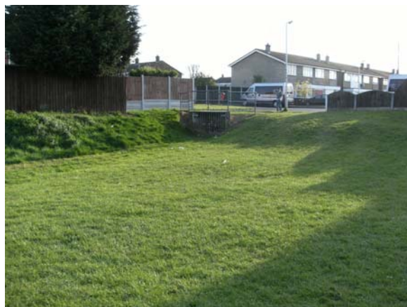
Figure 10-4: Albany Road, Flood Storage Area, Wickford
