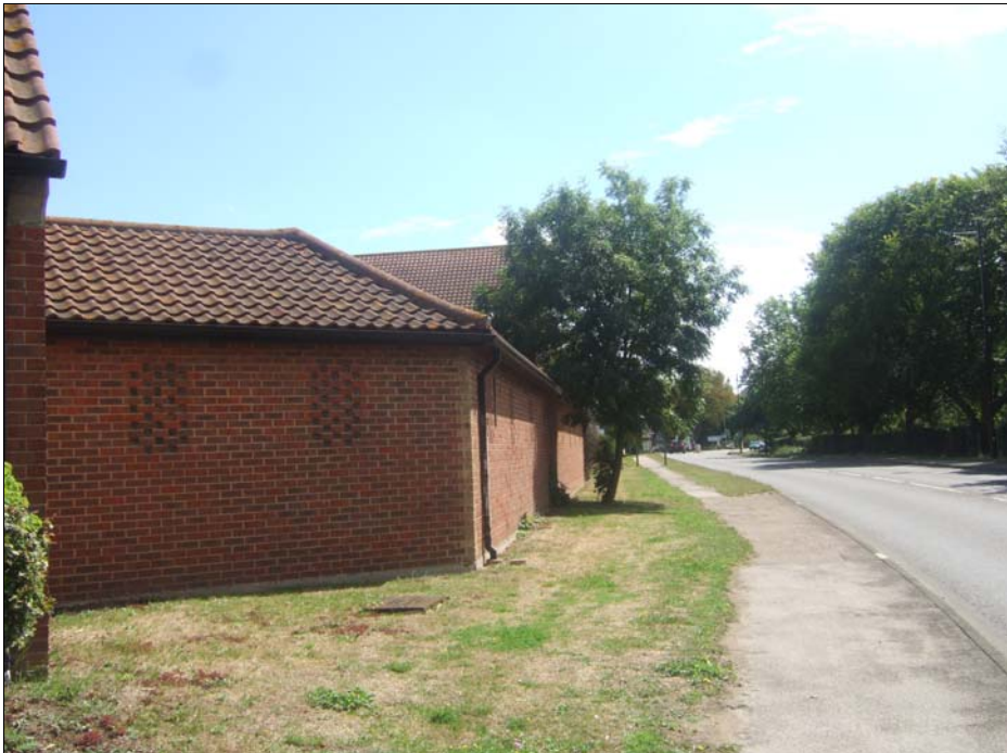
View along Bradley Way
