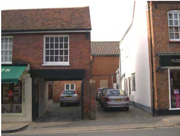
Fig. 26 South Street, carriage arch on the north side of no. 8.
