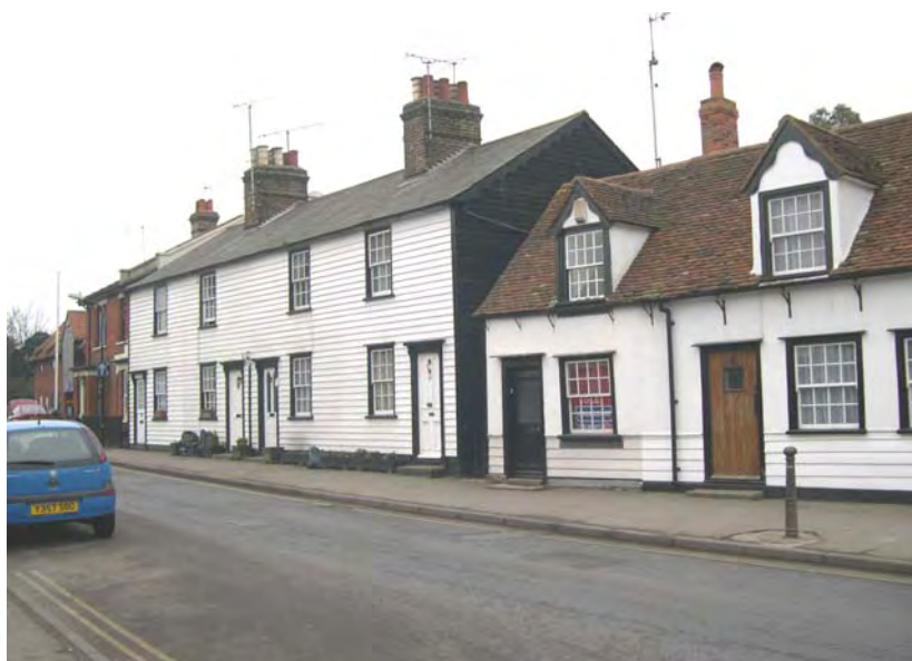
Fig. 55 Weir Pond Road, cottages at the west end (nos 6-16).
