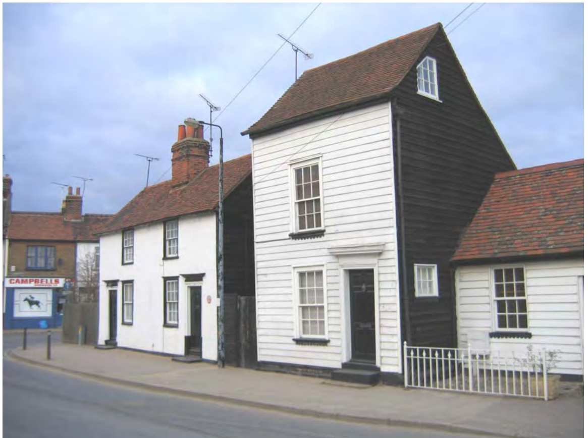
Fig. 10 North Street, no. 36, typical weatherboarding and black and white painted joinery. Nos 38-40 have a rendered or Roman cement painted façade, lined out in imitation of masonry.
