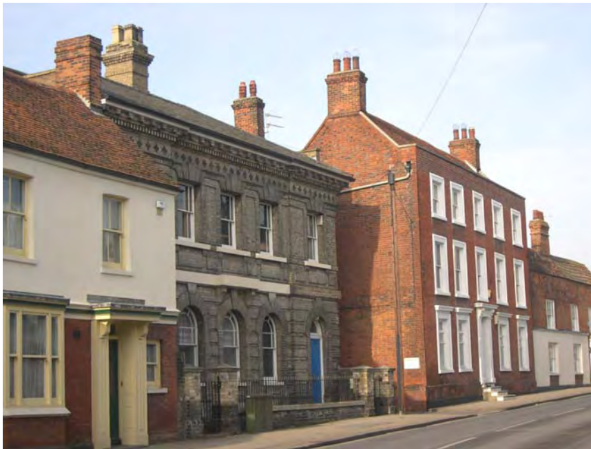
Fig. 28 South Street, no. 22 and the Masonic Hall, formerly the County Court.
