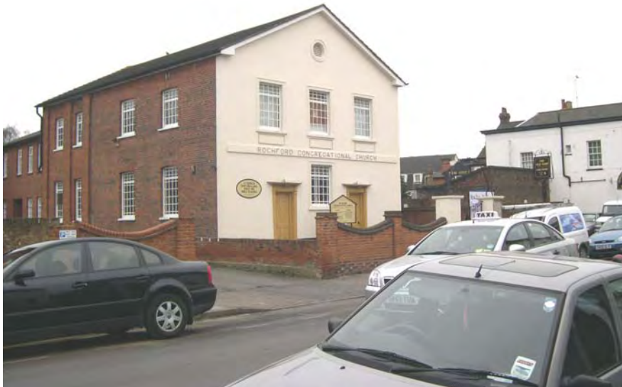
Fig. 53 North Street, the Congregational chapel.
