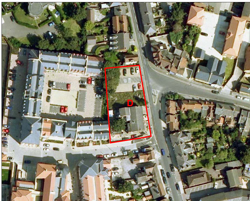
Aerial view of Site D
