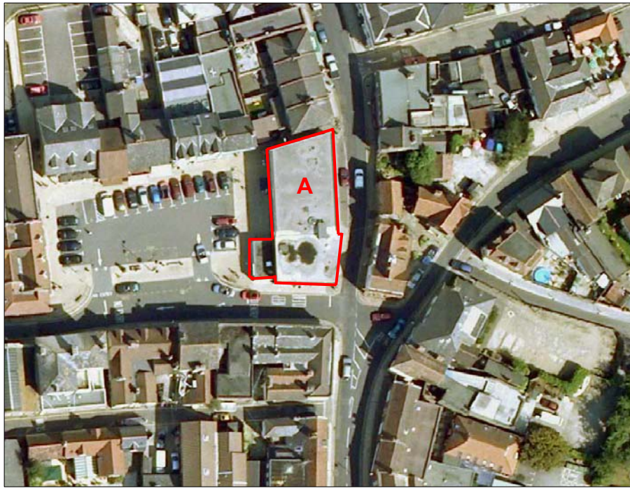
Aerial view of Site A – Eastern Side of the Market Square
