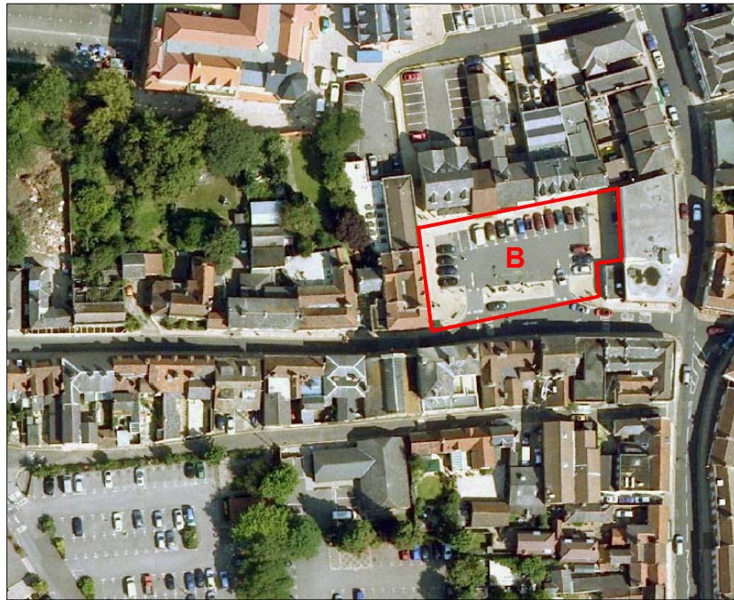
Aerial View of Site B –Market Square
