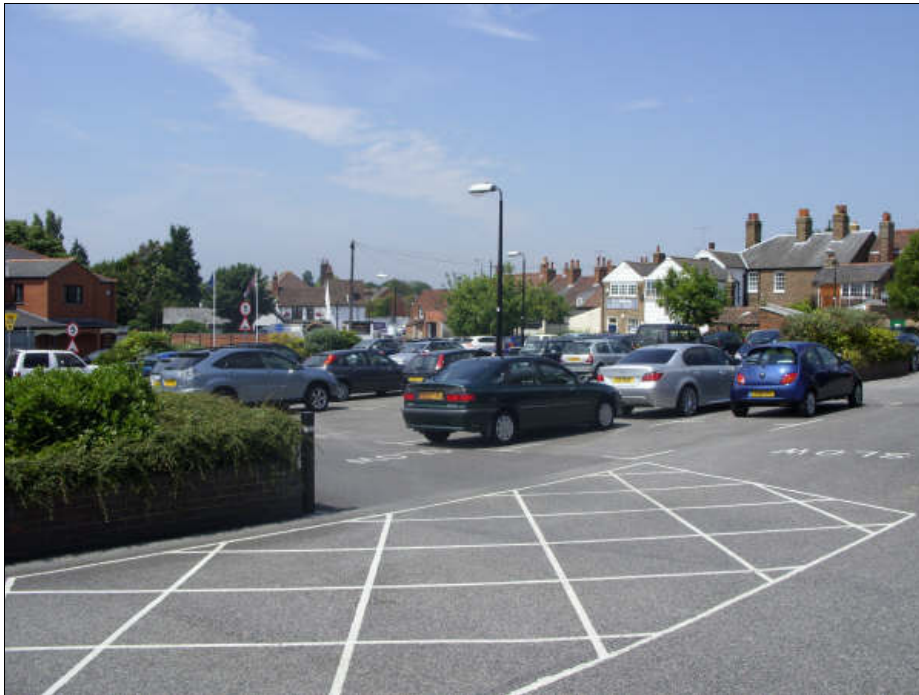
Back Lane Car Park
