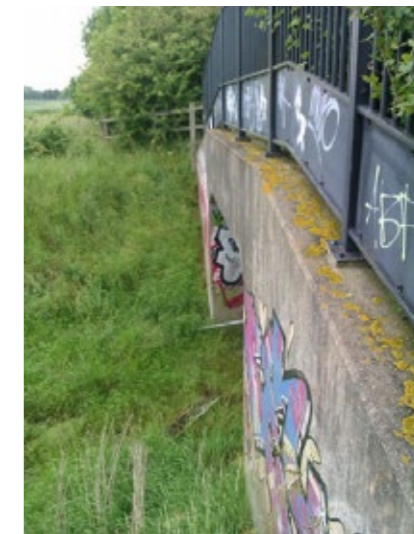
View of western access to Butterley Bridge
