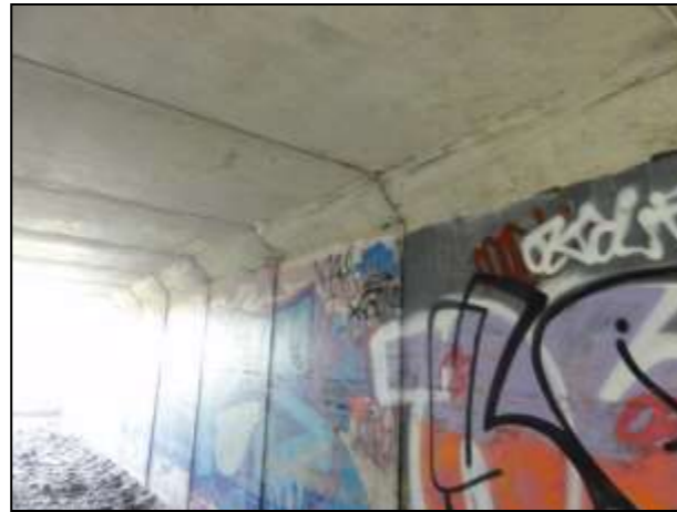
Photograph 17: Ceiling of the structure
