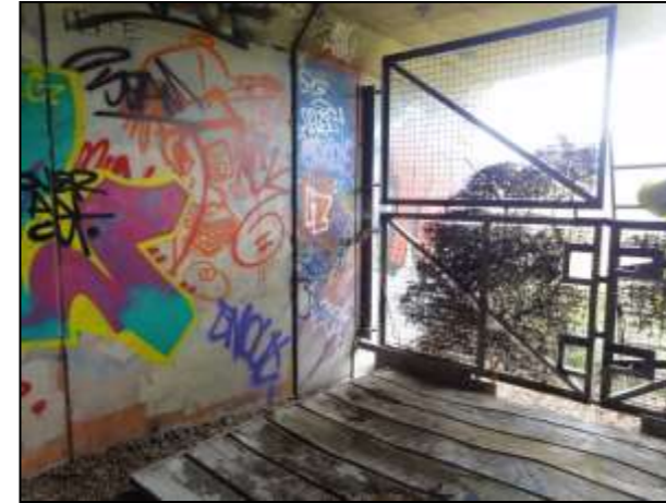
Photograph 12: West gate entrance
