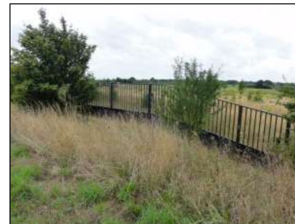
Photograph 5: Vehicle barrier from the road side
