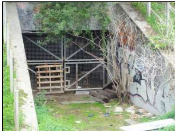
Photograph 11: Eastern wing walls
