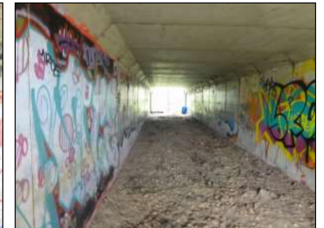
Photograph 15: General condition of the structure
