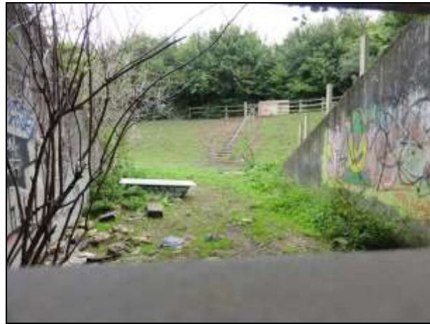
Photograph 9: Steps down to pumps
