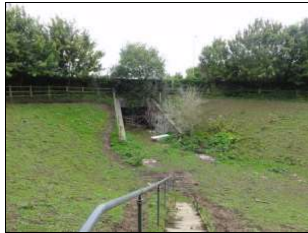
Photograph 10: Pump access chambers
