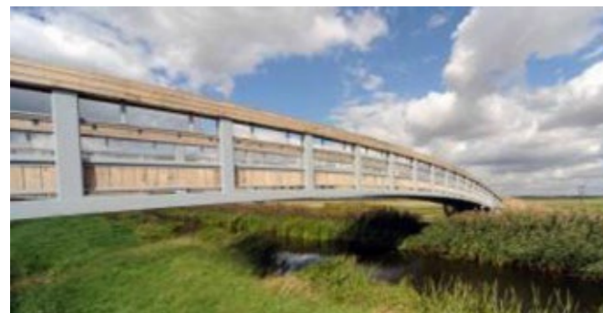
Reach Lode river crossing, Cambridgeshire
