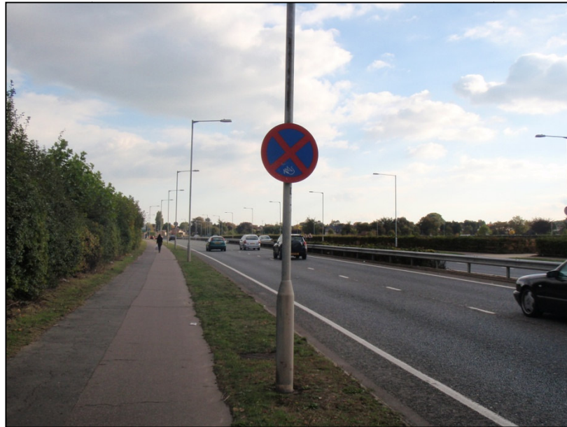
Figure 3.6 – B1013 Nestuda Way southbound carriageway
