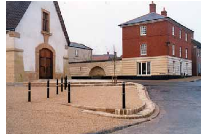
Shallow steps mediating height difference at Poundbury
