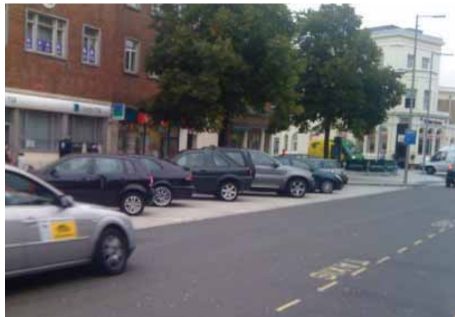
Echelon Parking at London Road, Southampton
