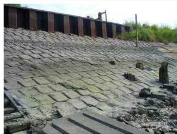
ROC07 Block revetment on earth embankment. ROC07 Steel capped revetment.
