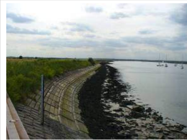
ROC07 Block revetment on earth embankment. ROC07 Steel capped revetment.
