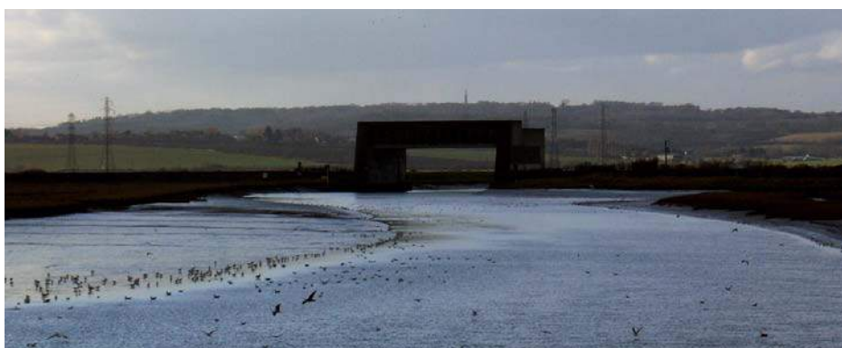
PLATE 6-9 FOBBING HORSE BARRIER AT HOLEHAVEN, THURROCK
