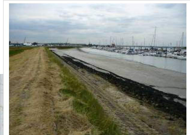
ROC05 Block revetment on earth embankment.
