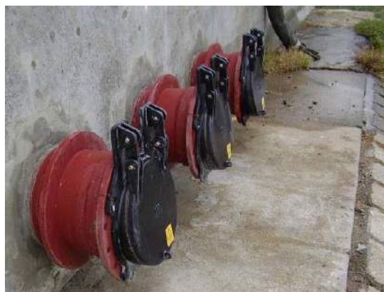
PLATE 6-8 EXAMPLES OF CULVERTS INSTALLED THROUGH FLOOD DEFENCES SHOWING TIDE FLAPPED OUTFALLS TO PREVENT A BACKWATER EFFECT DURING HIGH TIDE EVENTS
