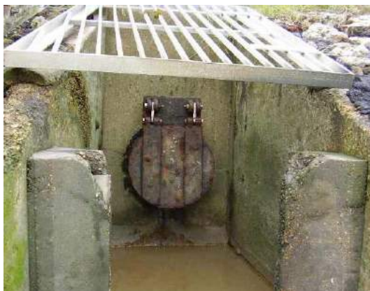
PLATE 6-8 EXAMPLES OF CULVERTS INSTALLED THROUGH FLOOD DEFENCES SHOWING TIDE FLAPPED OUTFALLS TO PREVENT A BACKWATER EFFECT DURING HIGH TIDE EVENTS
