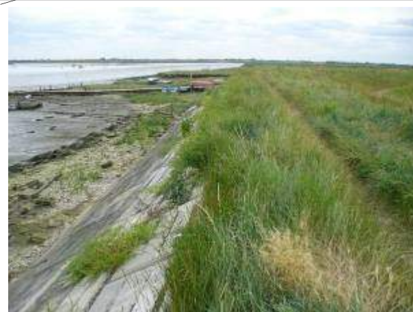
ROC04 Block revetment on earth embankment.
