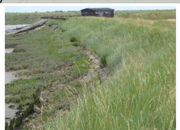
ROC03 Block revetment on earth embankment.
