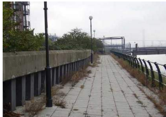
PLATE 6-6 EXAMPLE OF SHEET PILE WALL AS A SECONDARY FLOOD DEFENCE
