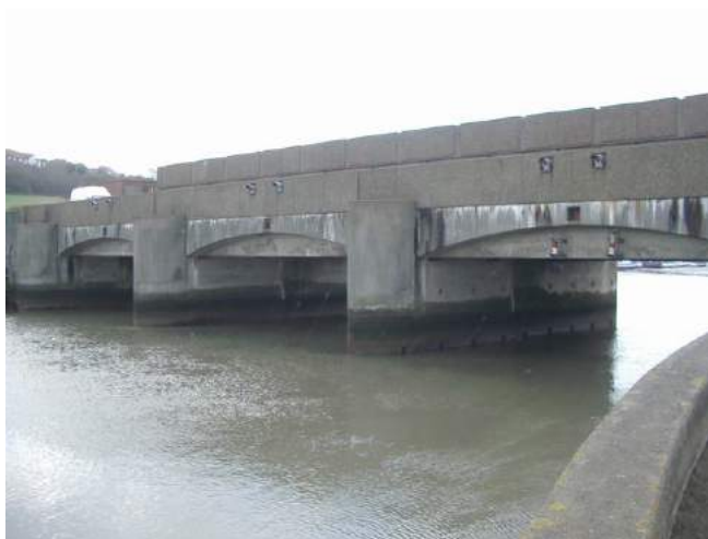
PLATE 6-10 BENFLEET BARRIER ACROSS BENFLEET CREEK AT CANVEY ISLAND.
