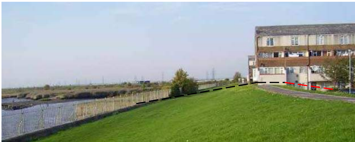
PLATE 6-2 EARTH BUND (RIVER THAMES, THURROCK) FORMING SECONDARY DEFENCE BEHIND CONCRETE DEFENCE WALL. THE CREST OF THE EARTH BUND IS UTILISED AS A RECREATIONAL FOOTPATH.
