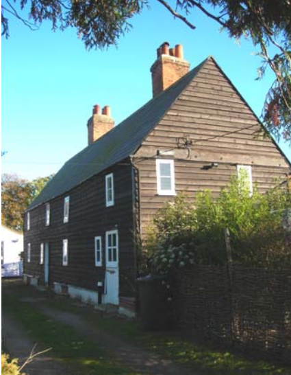
Fig. 35 Barn Row, north side.
