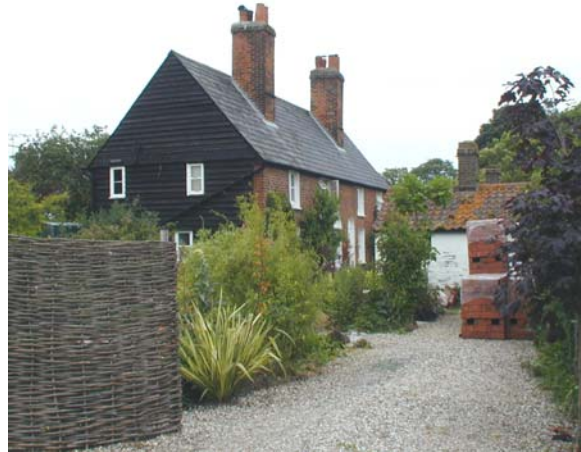
Fig. 36 Barn Row, south side, with pantiled wash house.
