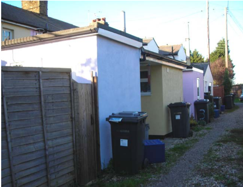
Fig. 38 Rear of Shop Row.
