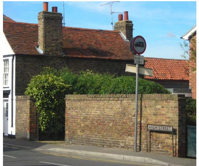
Fig. 23 Stock brick boundary wall, 2a High Street.
