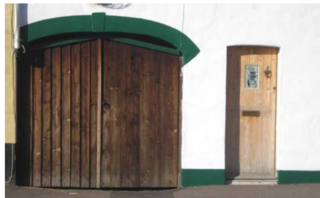
Fig. 25 Carriage arch, Prospect Cottages.
