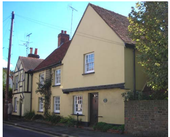
Fig. 42 Anchor Cottage, 17 High Street.
