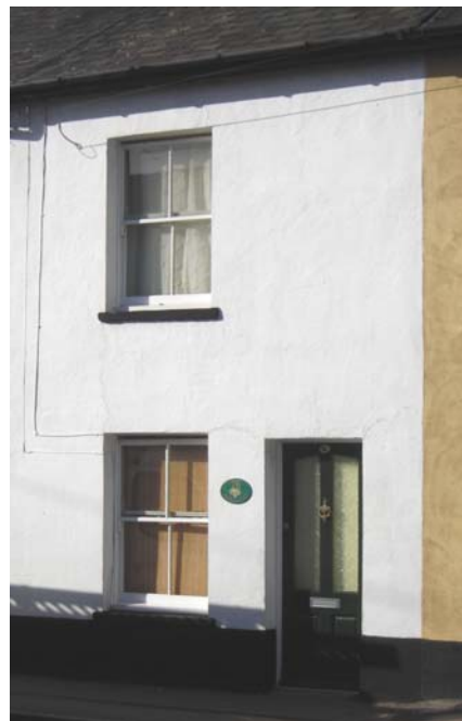
Fig. 22 Simple Victorian terrace façade, no. 76 High Street.
