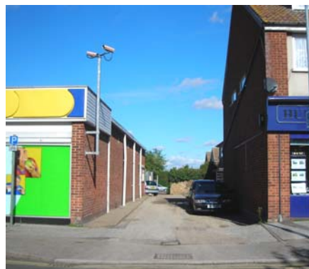
Fig. 83 Rear access between the Co-op and 20 High Street.
