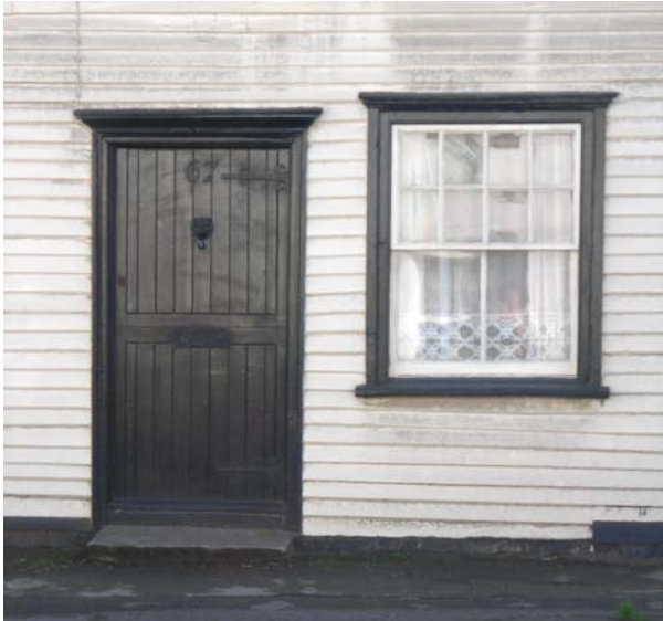
Fig. 20 Weatherboard and simple architraves, No. 67 High Street.
