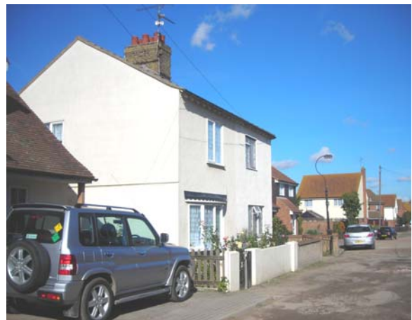
Fig. 49 Nos 3, 5 North Street.
