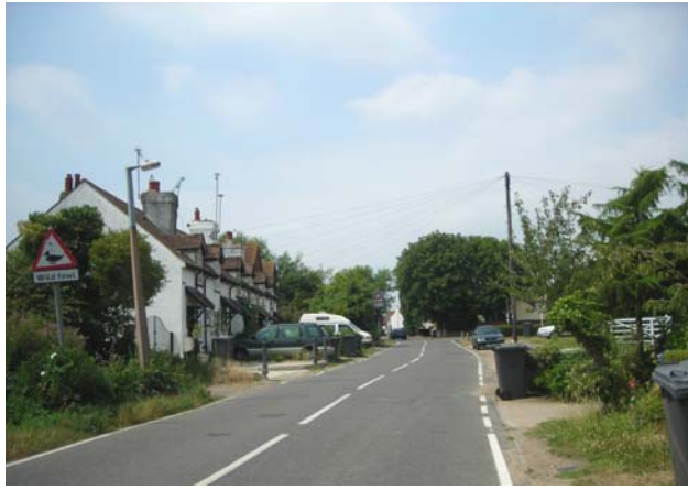
Fig. 12 Lambourne Hall Road.
