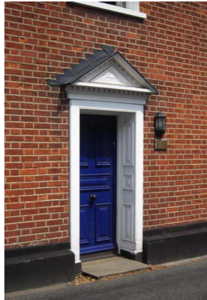
Fig. 24 Old Post Office.
