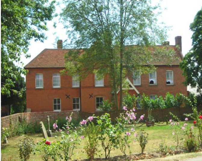
Fig. 20 The Vicarage viewed over the churchyard boundary wall.
