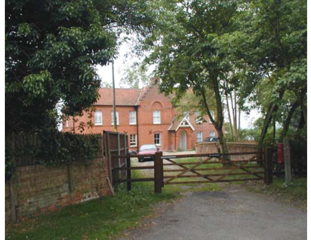
Fig. 13 View from the High Street to The Vicarage.
