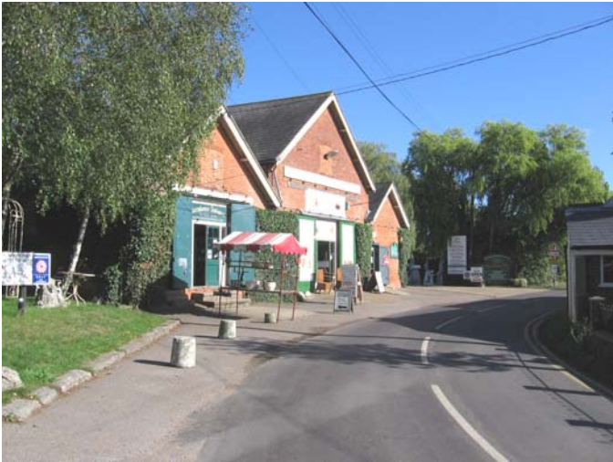
Fig.32 Muggeridge Farm barn.
