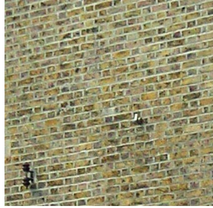
Fig. 15 Natural colour variation in 19th century yellow stock bricks on the old tide mill.
