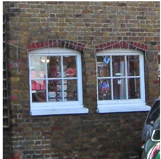
Fig. 17 Horizontally proportioned windows with cambered brick arches and painted timber joinery adjacent to the old tide mill.
