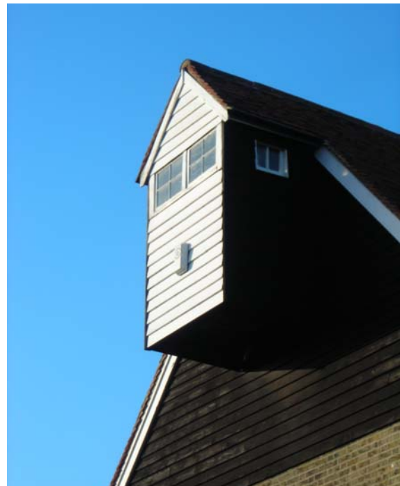
Fig. 14 Weatherboarded lucam on the old tide mill.
