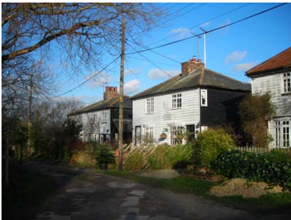
Fig. 50 Timber Wharf Cottages.
