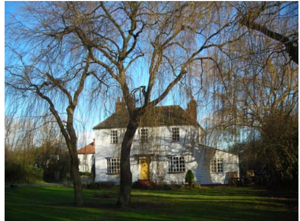
Fig. 49 No. 7 Timber Wharf Cottages
