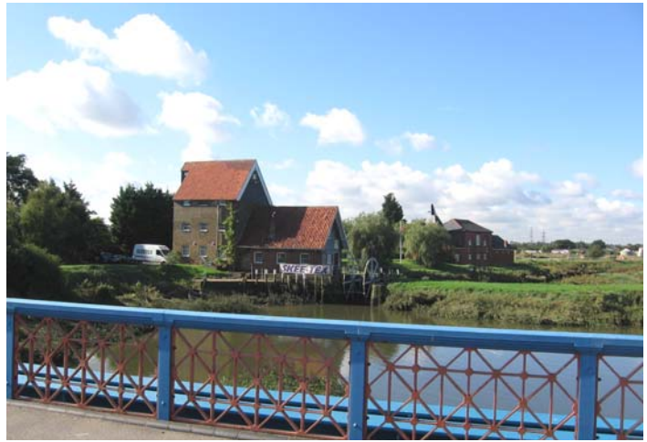
Fig. 21 View south from the bridge to the old tide mill, granary and drying kiln
