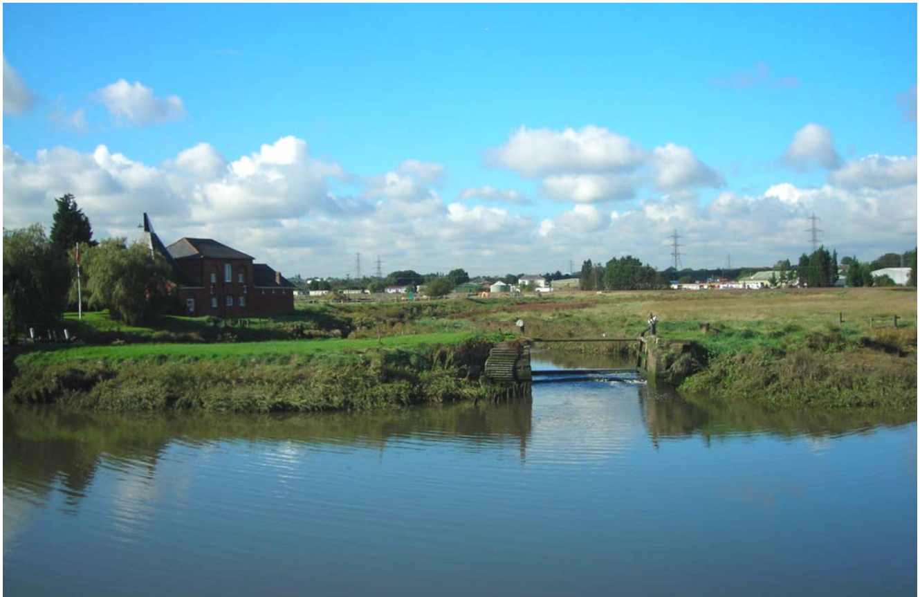
Fig. 11 View south from bridge with drying kiln and tide gates.
