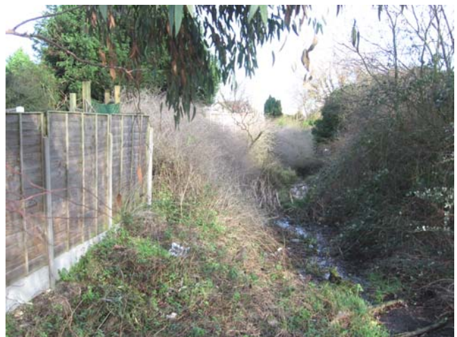
Fig. 24 Drainage channel to rear of Barge Inn.
