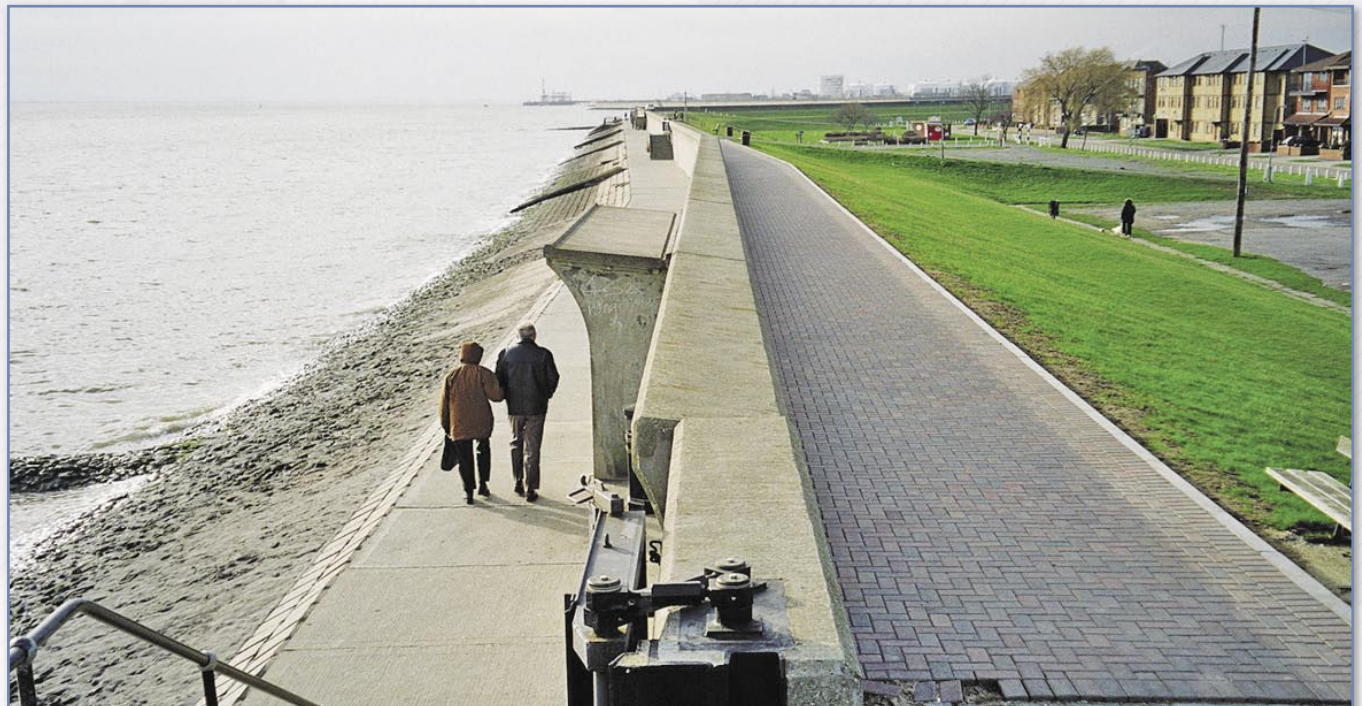
Sea wall at Canvey Island
