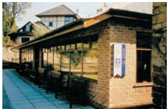
An urban bowls pavilion tucked into a narrow site. An eaves overhang provides some shelter along the green's frontage.
