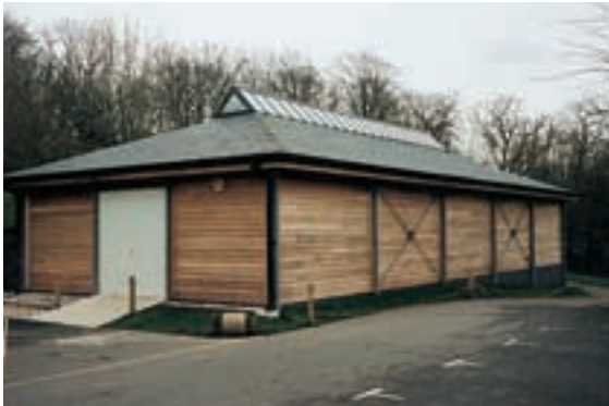
A rural storage building with exposed galvanised steel frame, cedar cladding and a spine roof-light; a low maintenance design concept equally applicable to a small clubhouse.
