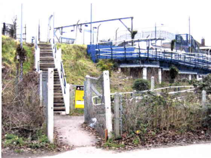
Fig. 20 Steps and ramp at the west access to Rochford station.
