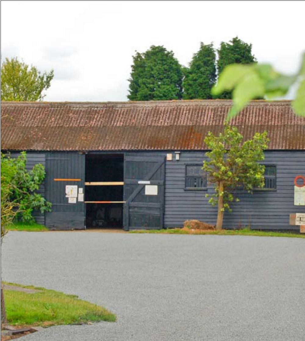
Tithe Barn is a typical example of an Essex clapperboard barn
