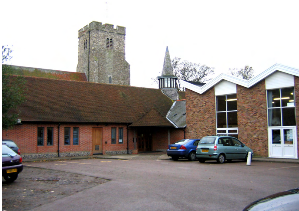
Fig. 22 The extension to Holy Trinity church.
