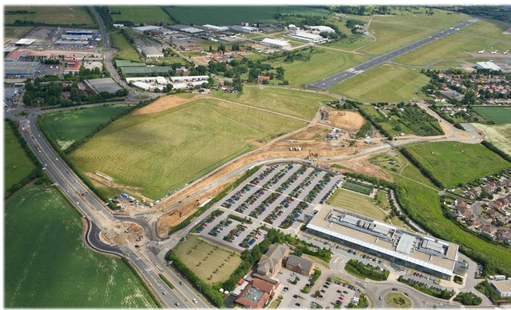
New link road under construction
