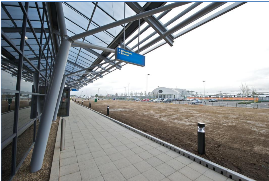
Terminal canopy providing weather protection
