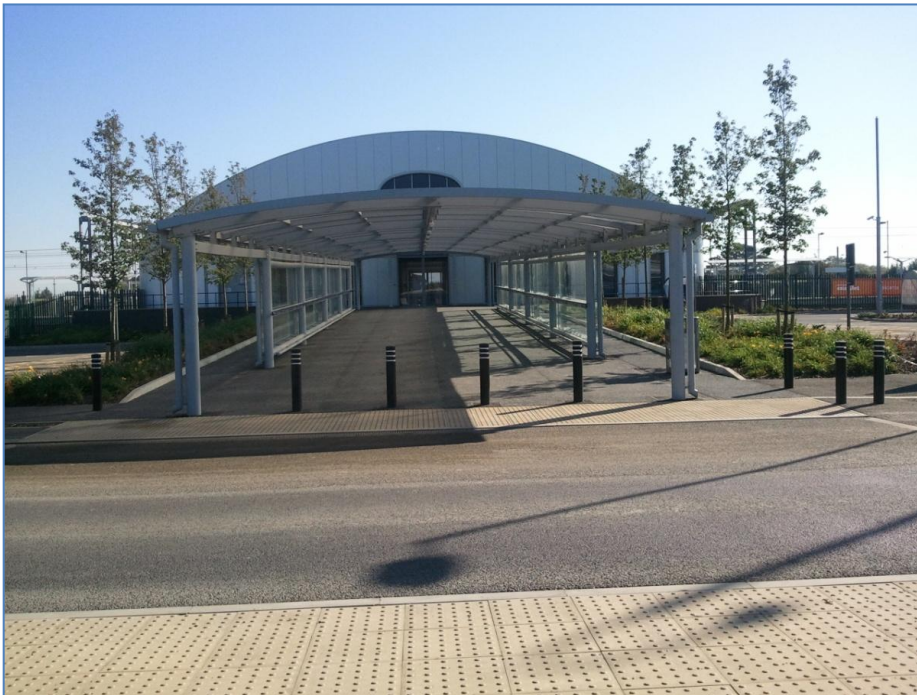
Tactile paving and ramp between terminal and station
